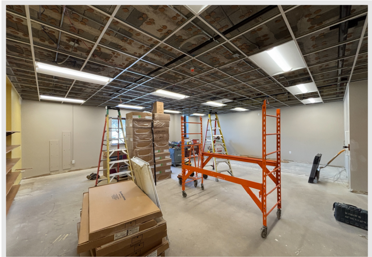
Ceiling grid/borders fully installed along with new light fixtures shining bright in the Second-Floor 3 rd Grade Classroom!
