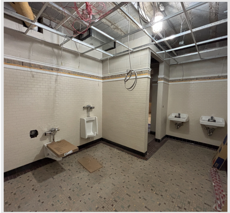
Floor and wall tile finished in the First-Floor Boys Restroom along with new plumbing fixtures in place. This space is looking sharp!
